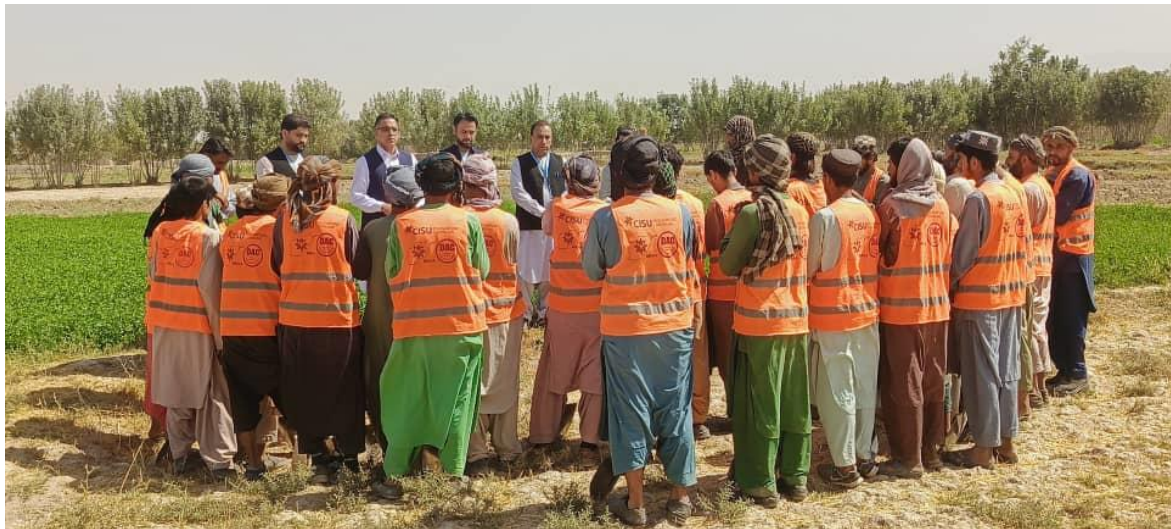
Workers are instructed regarding the canal's renovation
