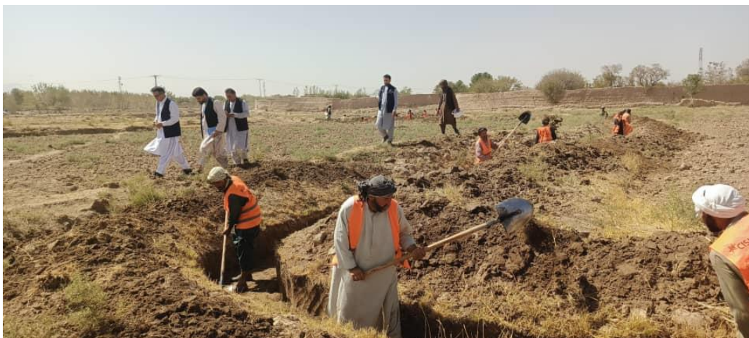
Work in progress – renovating the canals
